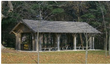
Allardale 32-person occupancy
